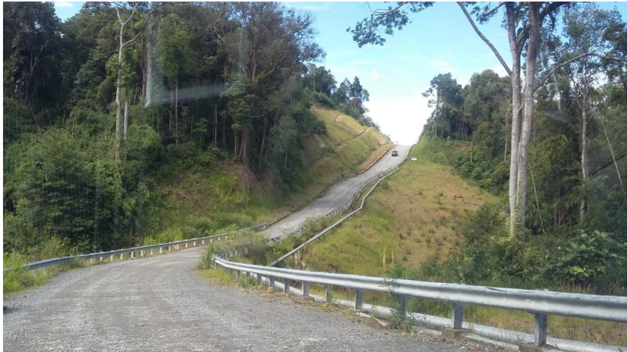
Figure 22. Sarulla project road showing wide cut-and-fill related clearing on either side of road for slope stabilization. Photo 2017 by E. Meijaard.
