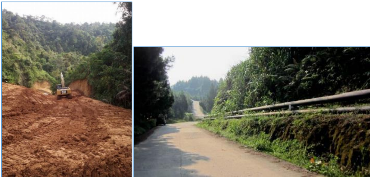
Figure 10. Environmental impacts depend strongly on the quality of project implementation and avoidance of damage. At 15-20 m, road clearings in Lumut Balai (left) are twice as wide as the 8 m wide roads in Gunung Salak (right) doubling deforestation, and increasing fragmentation and edge effects. Lumut Balai photo from internet search, and Salak photo 2017 by E. Meijaard
